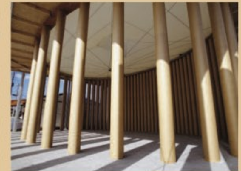
Top and above: Cardboard complexity – Shigeru Ban's emergency homes and temporary church pillars
