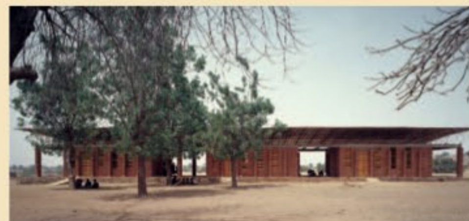
Opposite page and above: Deep in the Sahel – Francis Kéré's Gando school, under construction and complete
